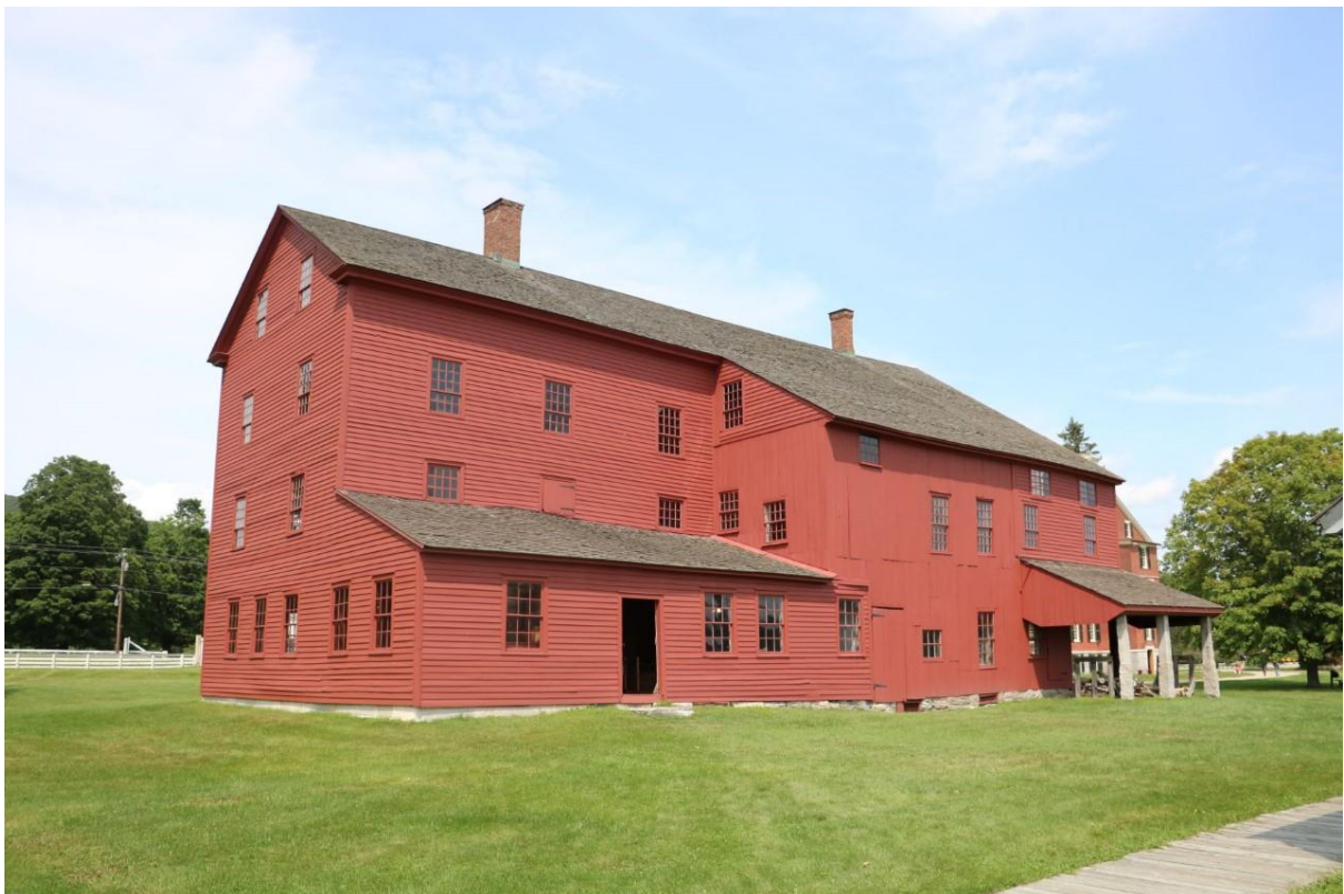
Hancock Shaker Village Workshop Building, Pittsfield, MA
