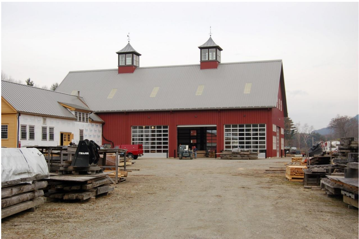
Timber Framing Company Dave Lanoue Workshop, MA
