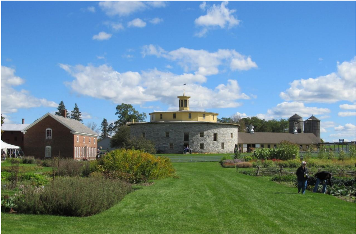
Hancock Shaker Village Barn, Pittsfield, MA
